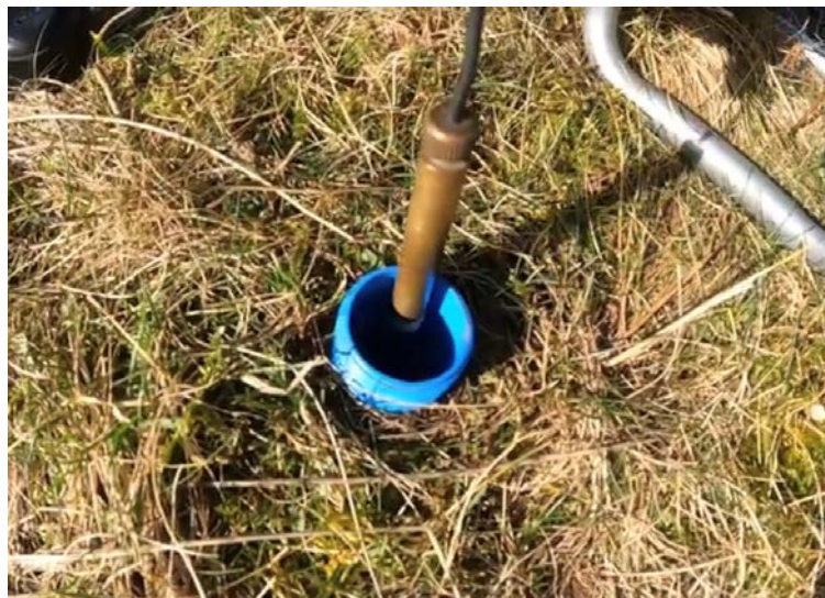
Figure 10. A dipwell installed at Ainsdale Sand Dunes National Nature Reserve.
