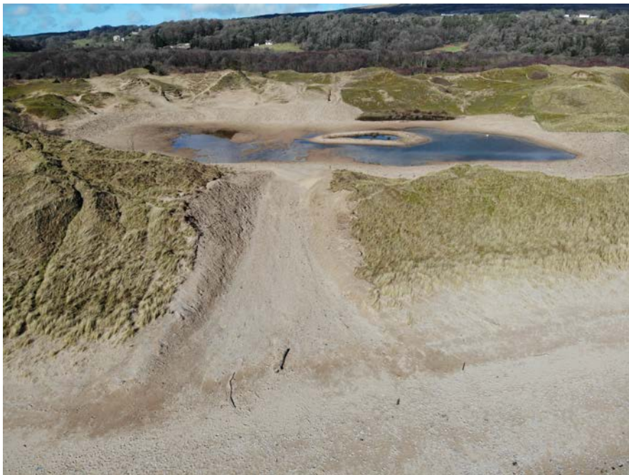
Figure 19. Aerial image of notch creation and turf stripping in foredune at Oxwich, January 2021. Photo, Natural Resources Wales.
